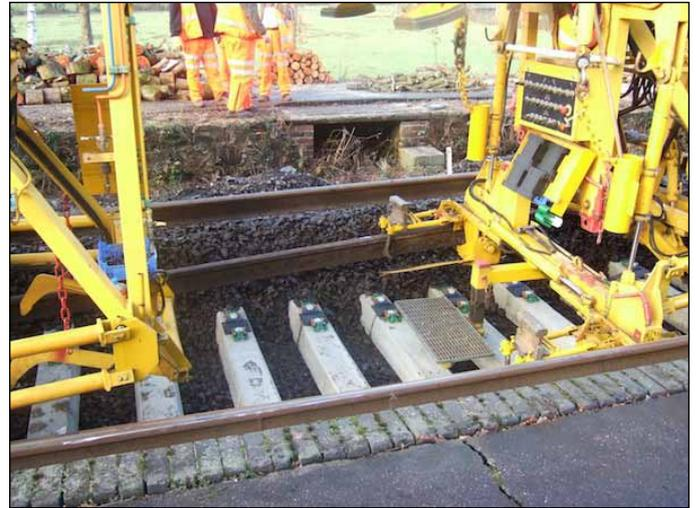
Figure 10. Replacement rail fed onto the newly-laid sleepers on 17 January.
