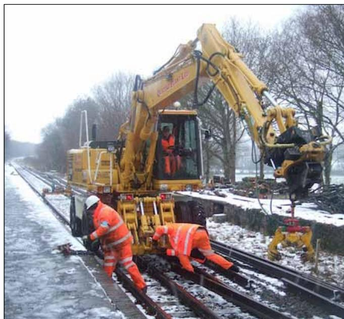
Figure 2. Positioning rail using one of the rail-mounted tractors on 12 January.
