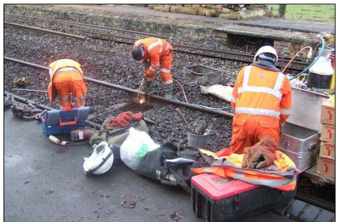
Figure 13. Preparing one of the rail joints for welding on 1 February.
