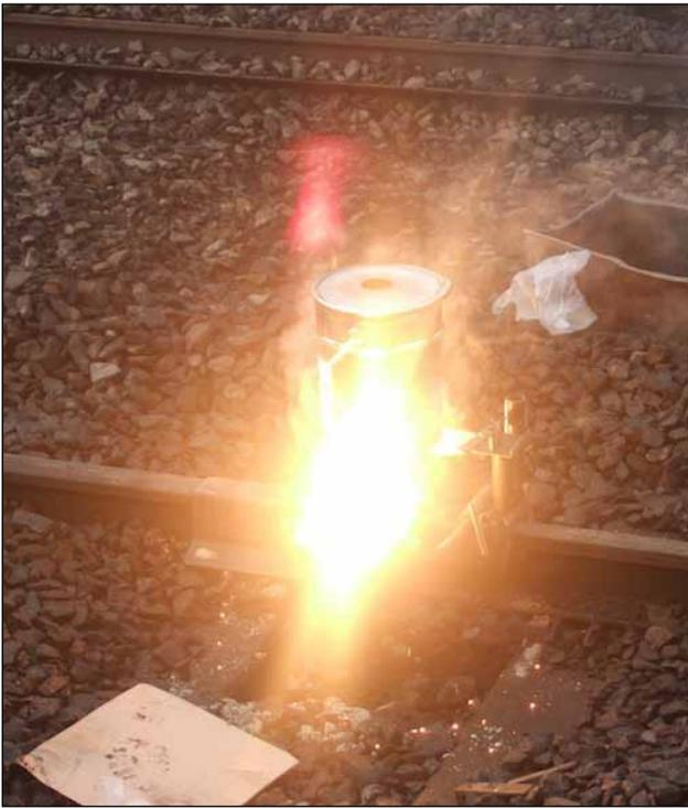
Figure 14. Thermite welding of the joint – fireworks at Bow!
