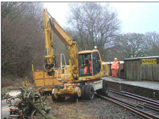
*Figure 4. Rail-tractor moves out of the way ready for arrival of the Tamper on 15 January.*
