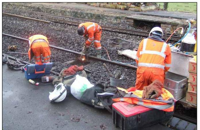
Figure 13. Preparing one of the rail joints for welding on 1 February.
