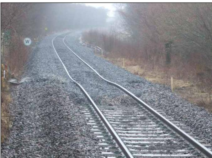
Figure 16. A minor hill in the track at the end of the day’s work on 23 February, before the HOBC restarted work.
