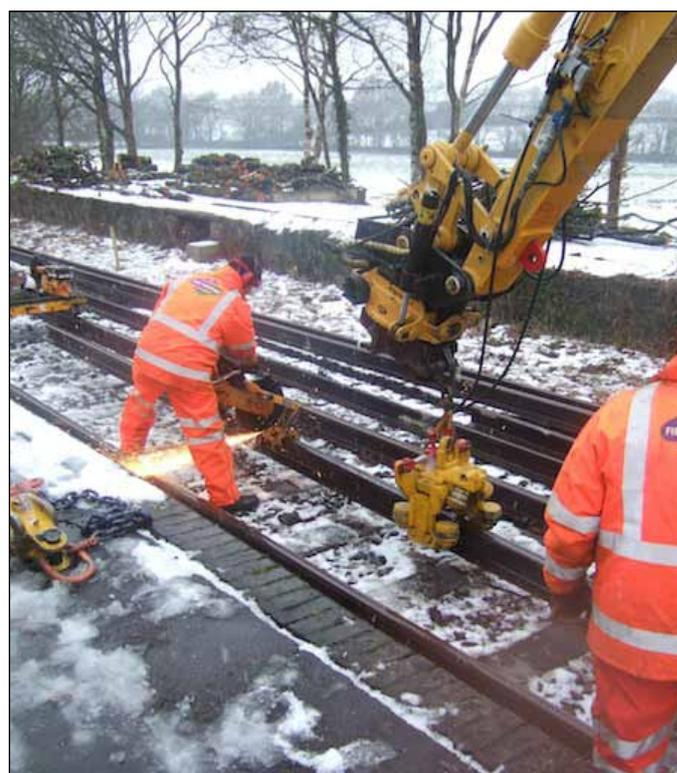
Figure 3. Cutting rail ends on 12 January; notice the rotten weather.
